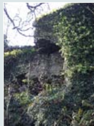
Significant loss of material to the internal face of section J
