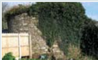
Heavy growth to external face of tower at Section L.
