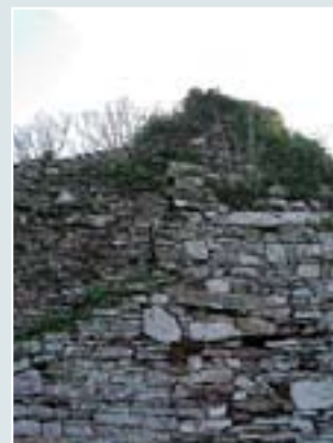
Bowing of external face of section J, note the open joints and heavy growth to wall
