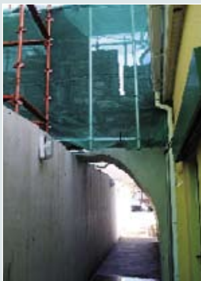
Hoarding protection to section R during works to adjacent court house.
