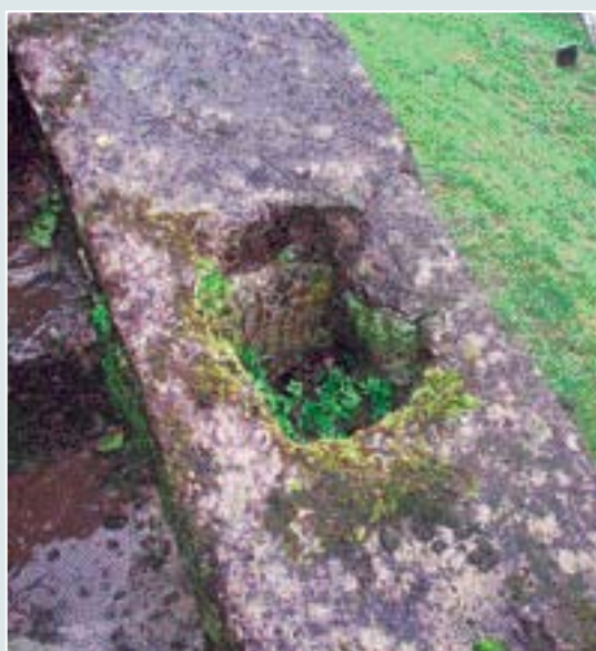
Socket from former railing to Section I, note plant growth to socket.
