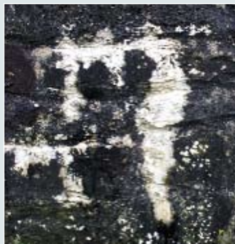
Lime leaching from internal face of section I.
