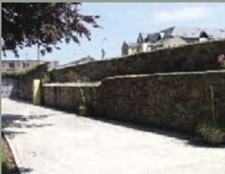
Plate 50. Section U – internal face with concrete capping of top of wall and wall walk
