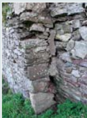
Detaching external face to section J, note the bowing of masonry.
