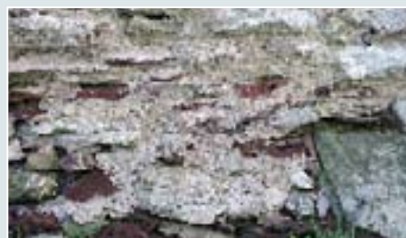
Poorly pointed stonework to external face of section J.
