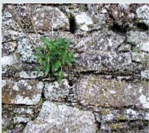
Lichen to stonework on external face of section J, note plant life to wall.
