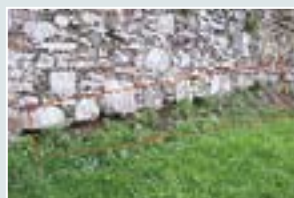
Missing stones to base of external face of section J.
