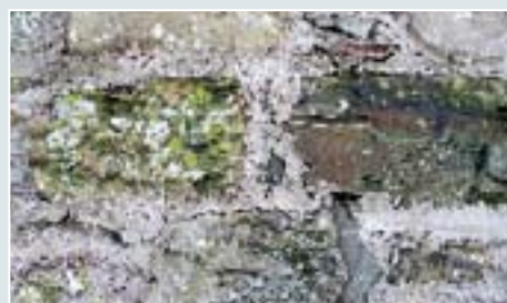
Stonework buttered with pointing material to external face of section J..
