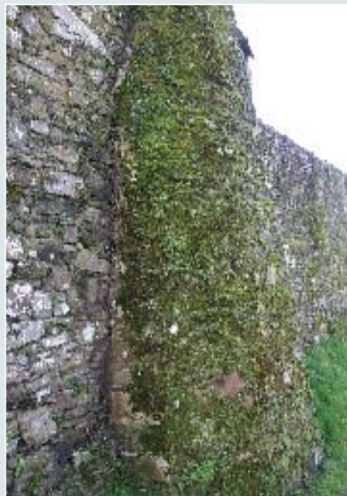
Heavy moss growth to battered internal face of Section I.
