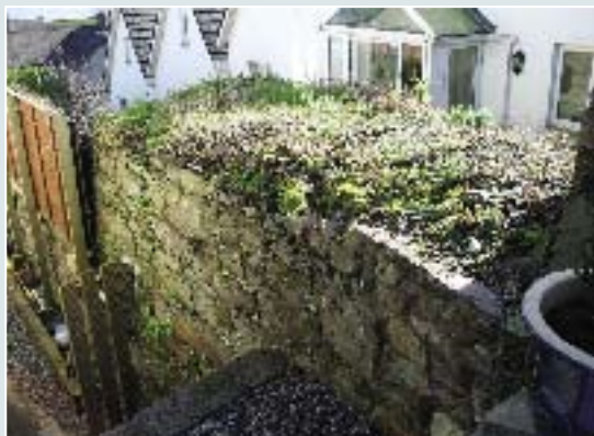
Plant life to cap of Section Q, note structures built up to wall.
