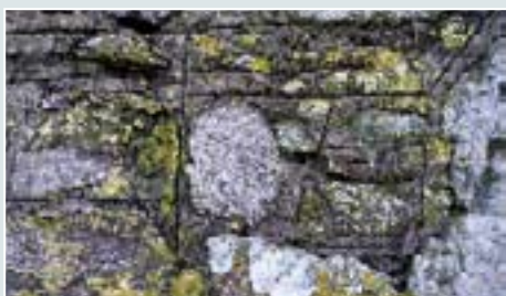
Cementitious pointing to external face of section J, note the poor pointing technique.
