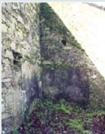
Scarring from former structure to internal face of Section J.
