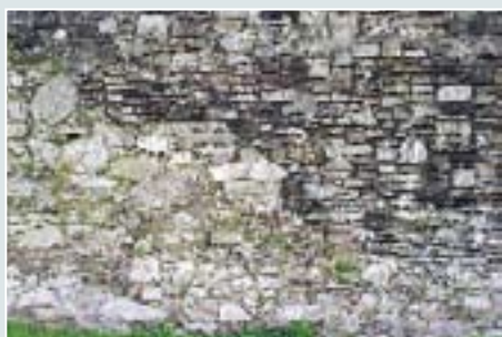
Junction of historic fabric and repair to external face of Section I, note the membrane lining to distinguish phases.
