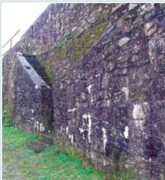
Missing railing to Section I.
