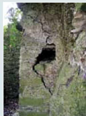
Substantial crack and void to internal face of section E
