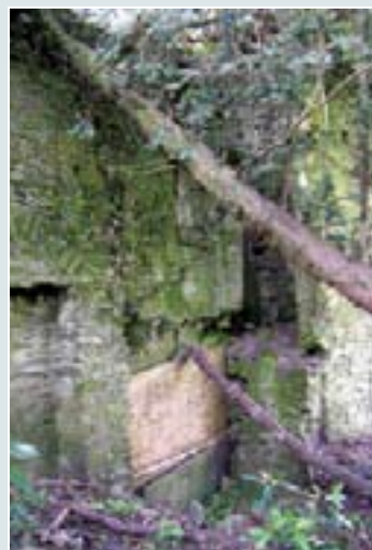
Fallen tree resting on head of wall at section E
