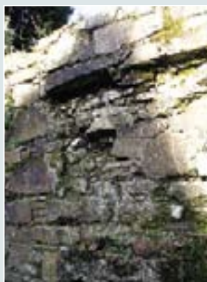
Voids to internal face of section F, where vegetation has been removed in recent times.
