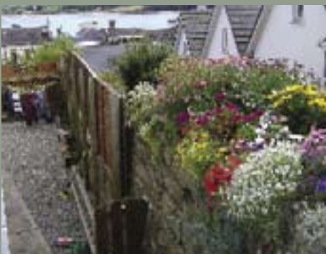
Plate 43. Section Q – vegetation growth on top of town wall. Note close proximity of recent developments
