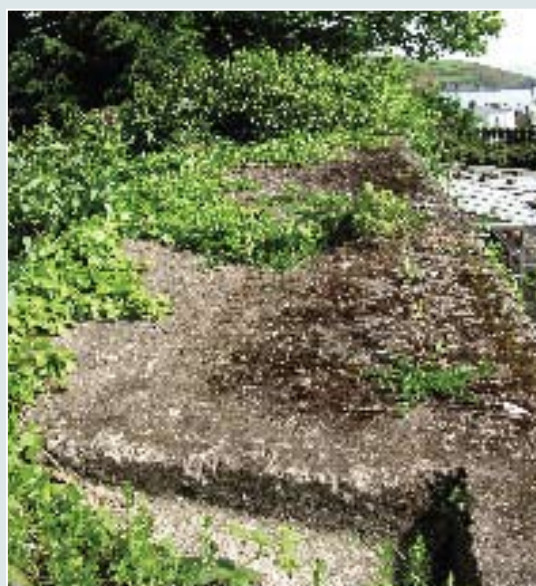
Cement capping to head of Section L.
