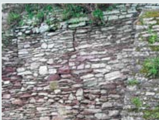
Open joints to external face of section K
