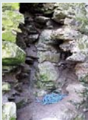
Large void to internal face of section J.
