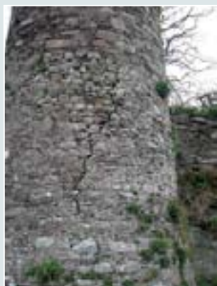
Structural cracking of external face of tower to section K.
