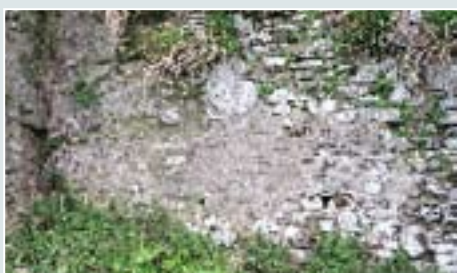
Cementitious pointing to external face of section K, note the poor pointing technique
