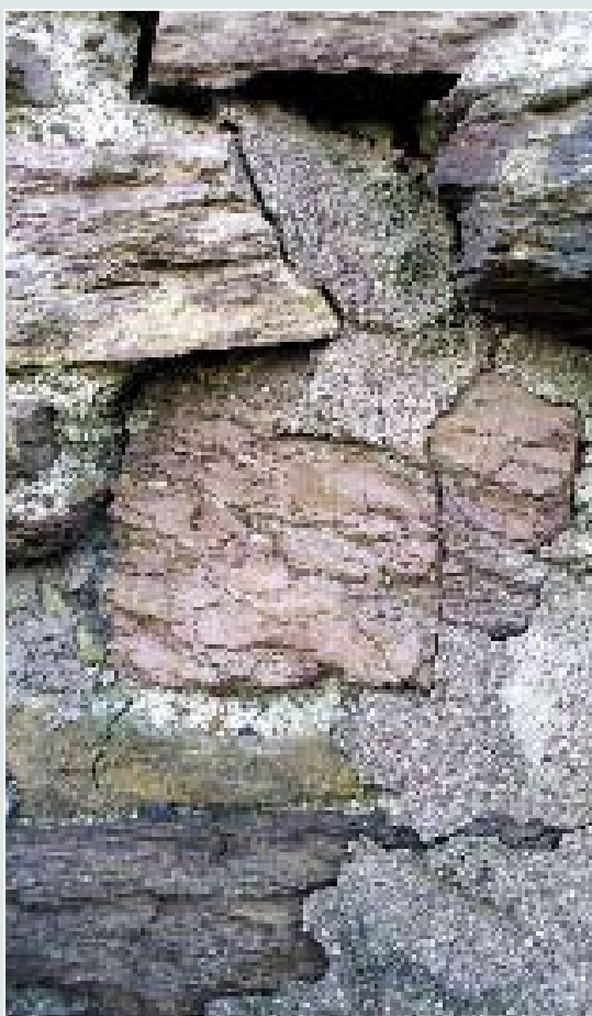
Fracturing of stone to external face of section I
