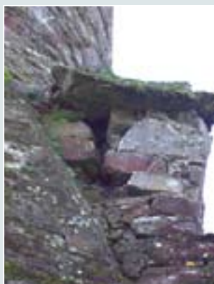
Structural cracking of internal face of section I adjacent breach in the wall.
