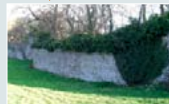
Heavy growth scaling the wall from the internal face of section K colonising the external face from the top down
