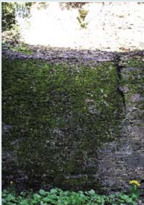
Heavy moss growth to sheltered internal face of Section F.
