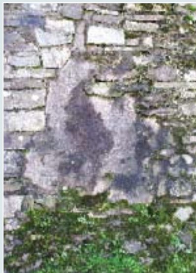
Cement repair of internal face of section I.
