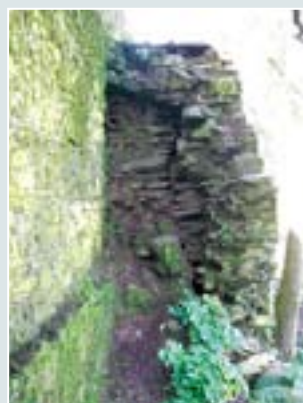
Loss of wall walk and exposed core to Section J
