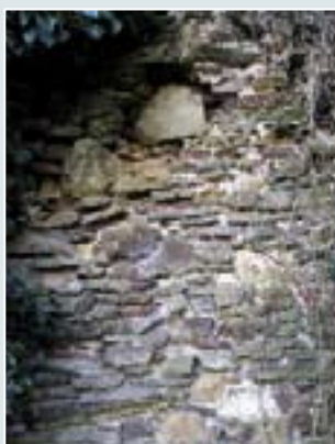
Voids to external face of section G, note the open joints to surrounding area
