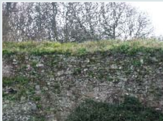
Plant life to cap of Section L.
