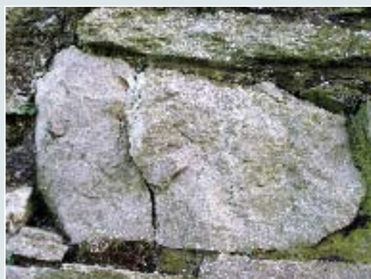
Fracturing of stone to external face of section I
