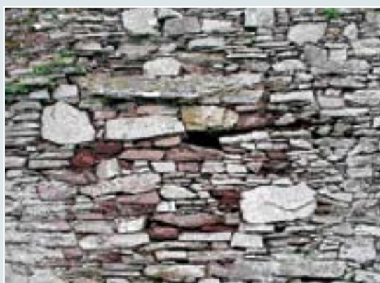
The continued action of rainwater has lead to the disintegration of pointing mortar to the external face of section J. Note plant life to adjacent areas.
