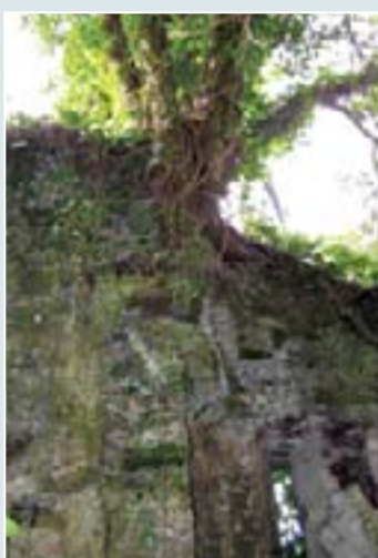
Mature tree growing from the wall head at section E.
