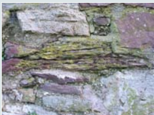
Cracking along bedding planes of stone to external face of section I.
