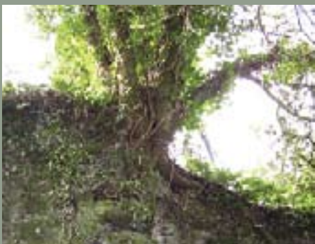
Plate 10. Section E – tree growth from top of wall
