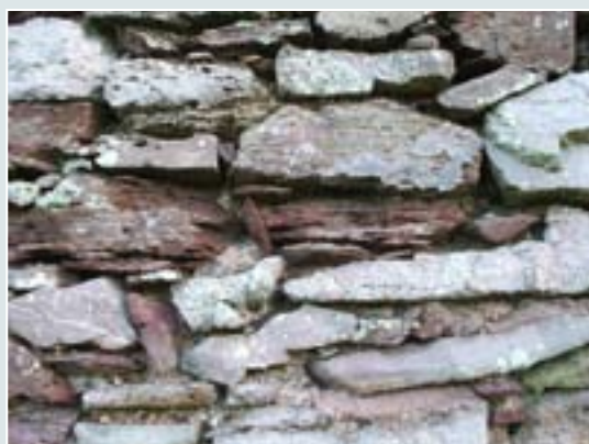
Cracking along bedding planes of stone to external face of section J, note the loss of pointing mortar to surrounding areas.
