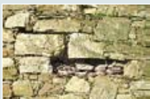
Voids to external face of section G, note the open joints to surrounding area
