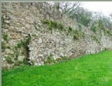
Plate 24. Section J – external face. Note line of vegetation along old top of wall
