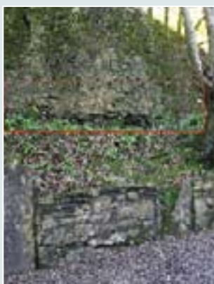
Missing stones to base of internal face of section F, note the heavy moss growth to sheltered areas.
