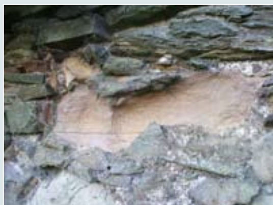
Significant dissolution of stone to external face of section G.
