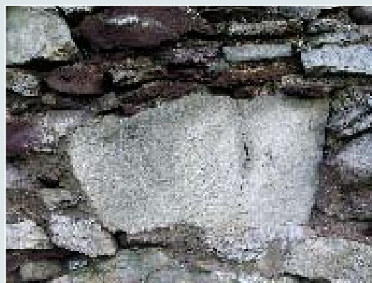
Fracturing of stone to external face of section J
