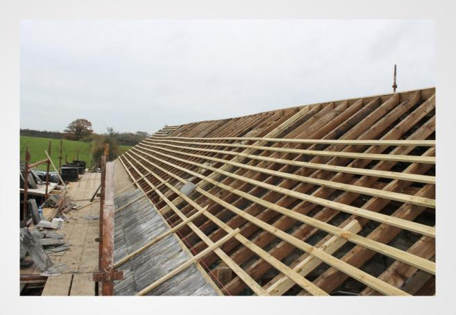
New battens on existing timbers. Some timbers spliced.
