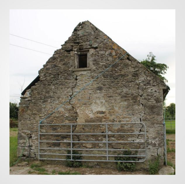
Cracks may no longer be opening up and can be stitched and filled.
