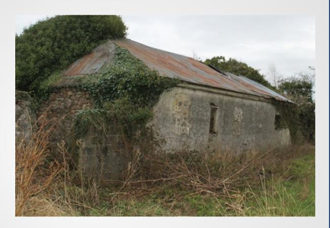
Significant rotation of rear wall. Ground conditions very poor in close proximity to Shannon River
