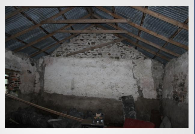
Undersized rafters and lack of adequate horizontal tie shall contribute to rotation of the walls.
