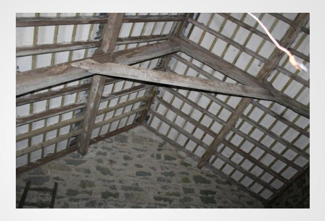
Provide lime parging to underside of slates. This provides additional protection water ingress and also resistance to wind suction.
