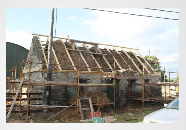
New Timbers constructed over existing so that ceiling could be maintained.
