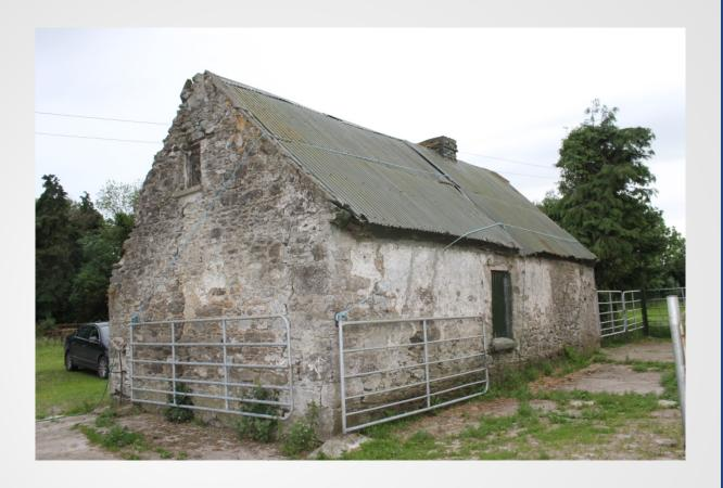
• When roof sheeting is excessively corroded, the only solution is to replace.
