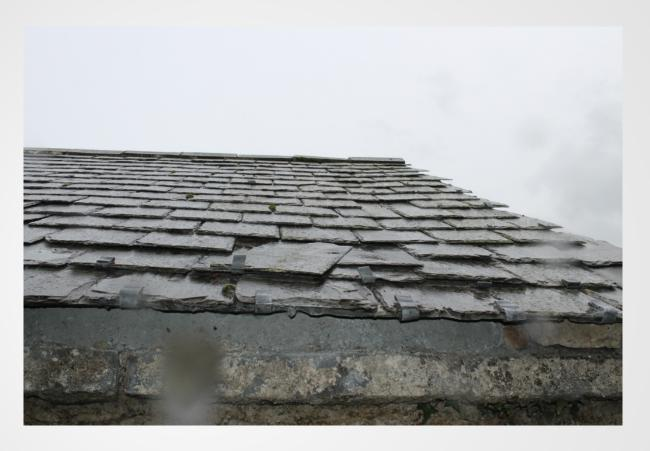
• When 25% - 30% of slates have slipped you should consider full re-slate of roof.
