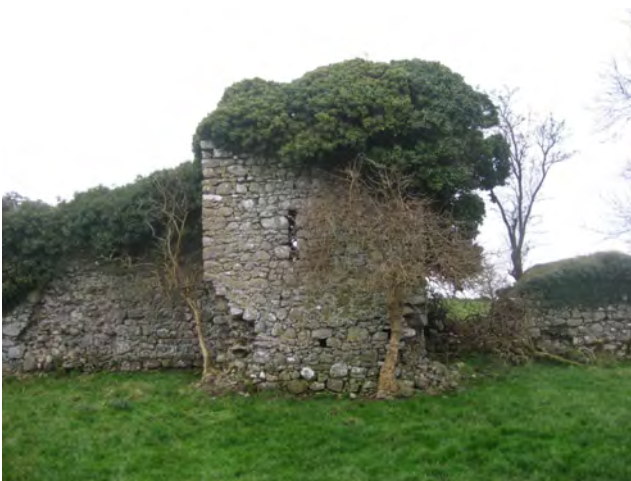
Figure 8.02 Loss of masonry at corners
