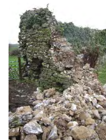
NORTH-EAST PIER OF GATEHOUSE FOLLOWING COLLAPSE
