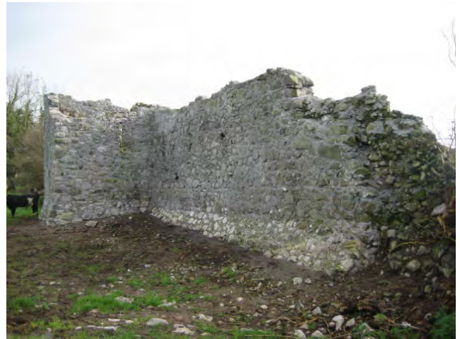
Figure 4.21 Stone course line in the wall adjacent to Tower Two
