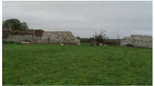
Figure 4.24 Wall loss at field gate opening
