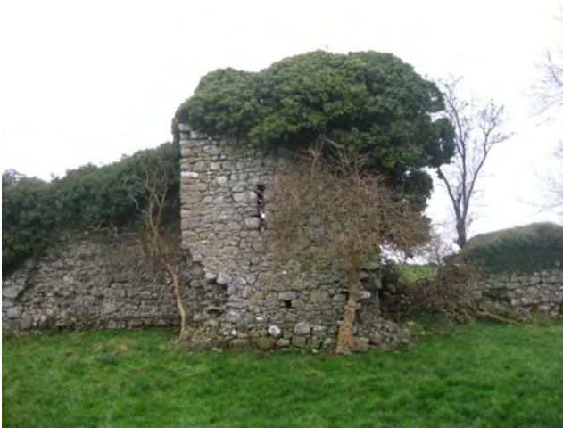
Figure 4.25 Tower Three prior to Conservation Works: The battered corners dangerously lost.
