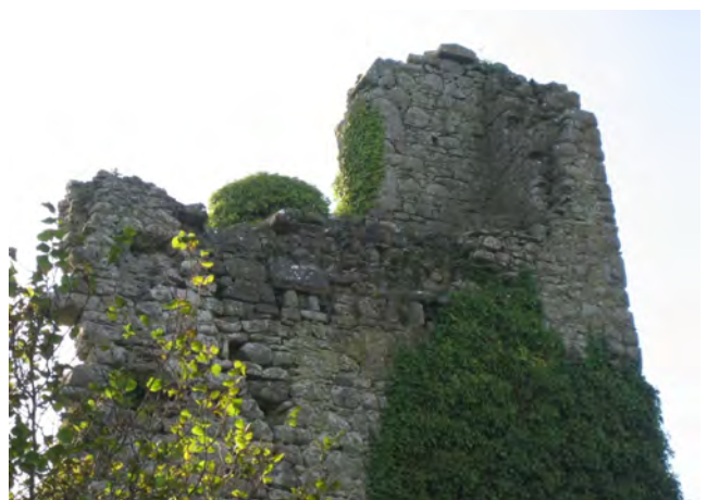
Figure 4.53 The highest section of Castle walls: A wealth of interesting masonry features, vulnerable wall heads and invasive plant growth.
