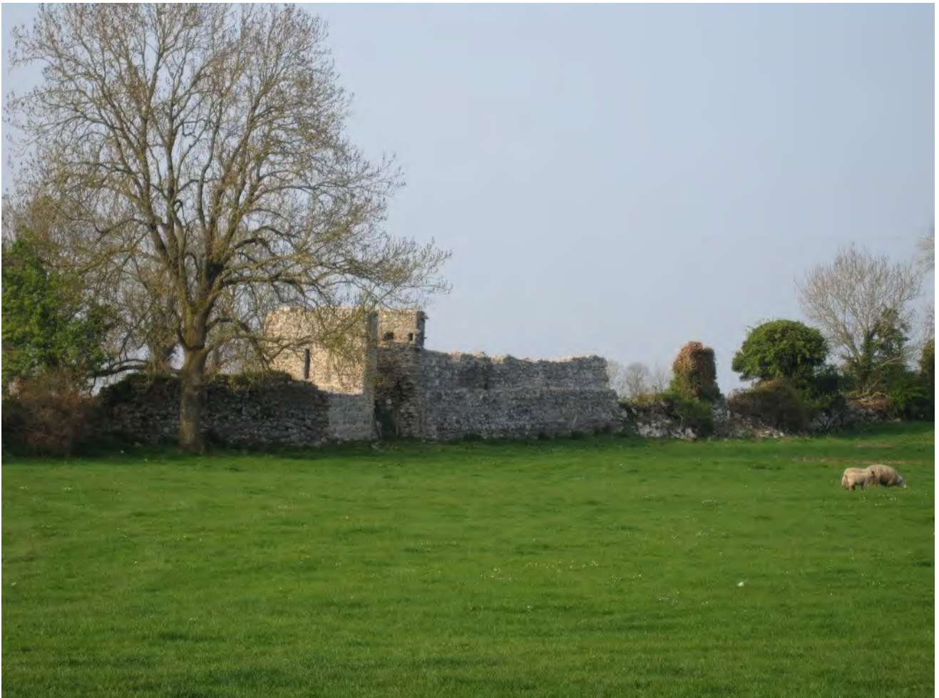
Figure 4.23 Tower Three, and adjacent wall. This illustrates the variation in condition of the surviving wall. The central section and Tower Three underwent emergency conservation works in 2009, and survive close to their original height, and have a wall walk ledge in the masonry. The length of wall immediately to the left (south west) survives to a reasonable height but is in need of stabilisation. Much of the wall to the right (north east) has largely fallen and has been seriously overrun and undermined by trees and ivy growth.
