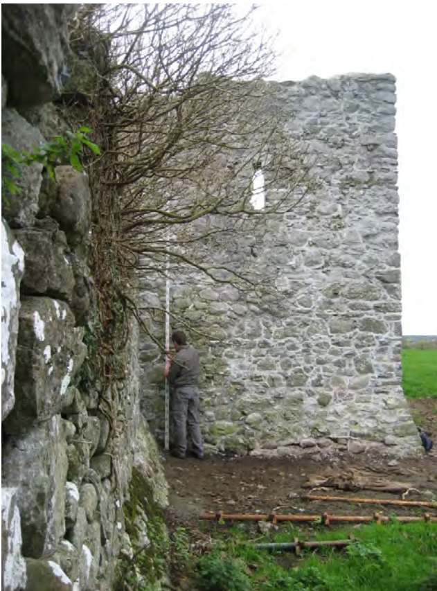
Figure 4.20 Battering at the base of Tower Two and adjacent wall
