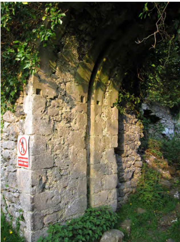
Figure 4.52 The Gate House into the Castle, Note the level of surviving fine detail and the invasive ivy growth and fallen masonry.
