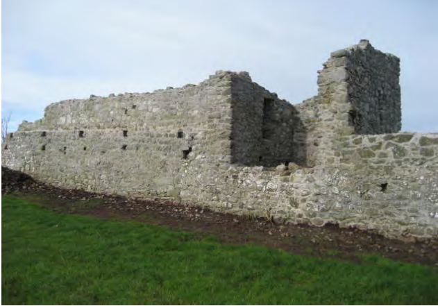
Figure 4.19 Putlogs below the wall walk ledge, adjacent to Tower Two
