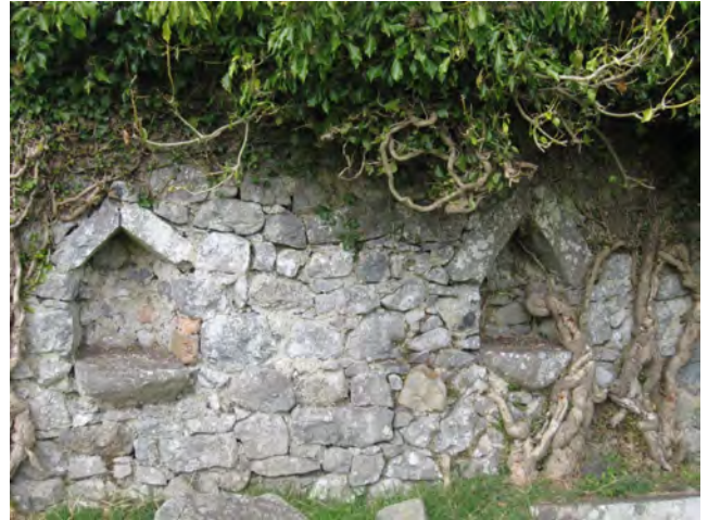
Figure 4.68 Bee-boles: note the ivy trunk penetrating the stonework in the bee-hole
