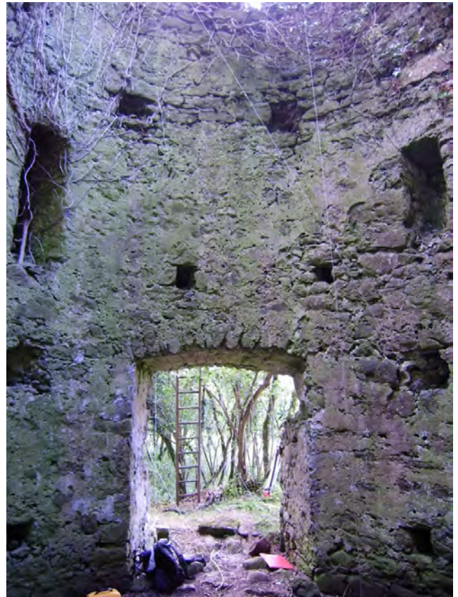
Figure 4.11 Masonry recesses and surviving plaster in the interior
