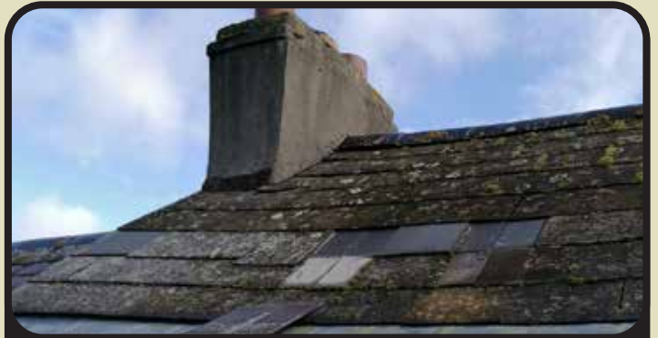
The missing slates, lack of adequate flashing around the chimney and loss of mortar between ridge tiles were causing several leaks in this roof.
