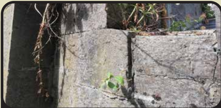
Inappropriate, and now cracking cement mortar being used on a stone wall will ultimately make a bad problem worse.
