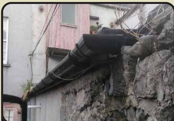
Clogged with vegetation at one end and with a clear gap at the other, this gutter is bringing water back into the building.
