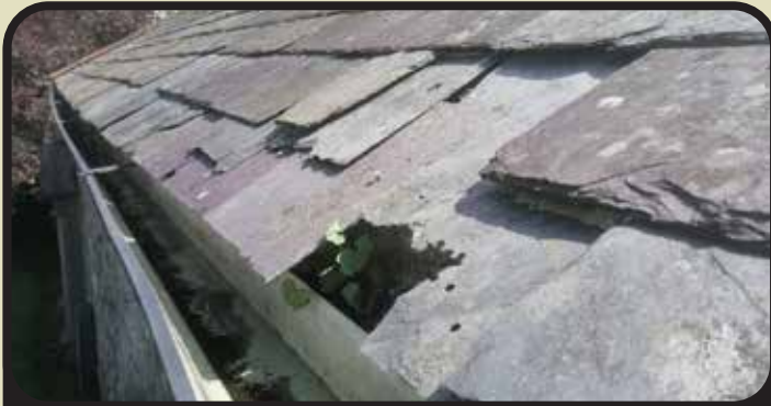
The missing and broken slates are causing water to run directly into building.
