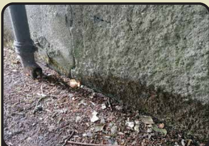
Water from this downpipe is being directed against a wall, causing it to be saturated.
