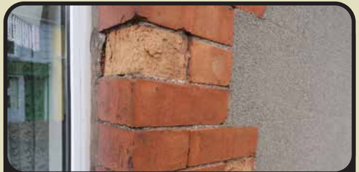
Although this image is of an early 20th century building, the hard cement pointing and render has forced the moisture in the wall to go through the softer brick rather than the supposedly sacrificial mortar and render.
