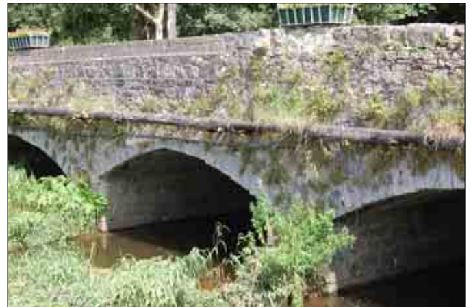
Arches of north face of bridge, looking south-east
