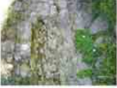
PHOTO 64 & 65. LOSS OF FACEWORK UP TO 350 THICKNESS LOST. CORE REVEALED. URGENT CONSOLIDATION REQUIRED.
