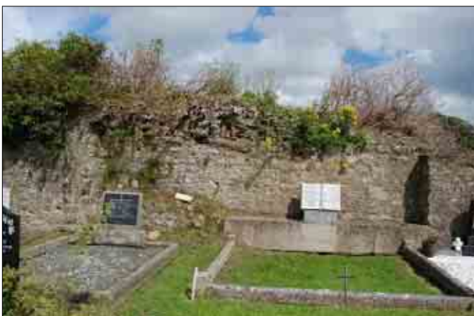
Interior side of east boundary wall, north end, looking east
