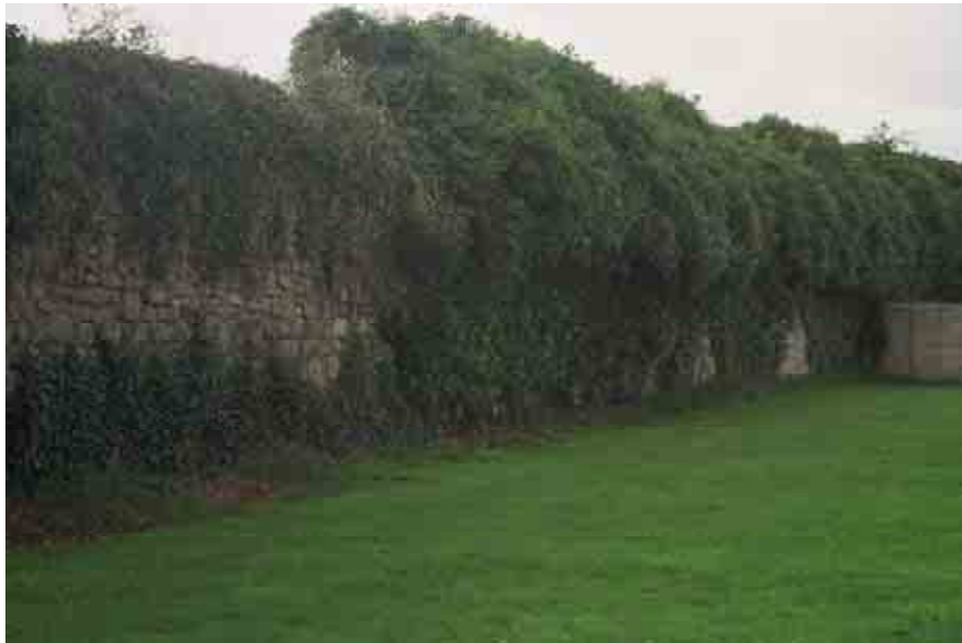
Plate 30: Internal west wall (courtesy of S. McCutcheon)
