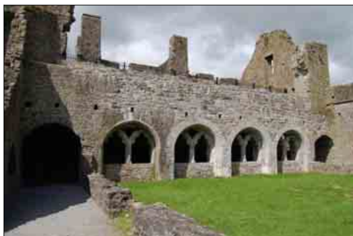
Detail of cloisters, looking north-east
