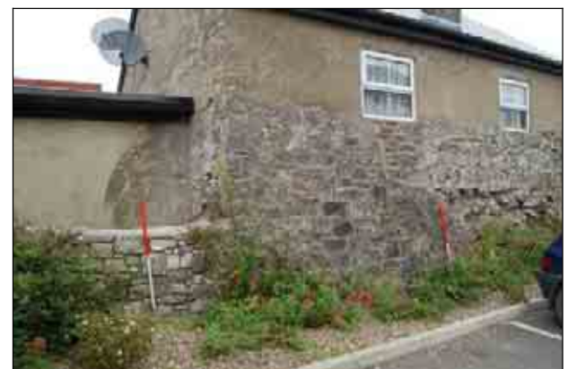
Exterior face of wall by house, looking north
