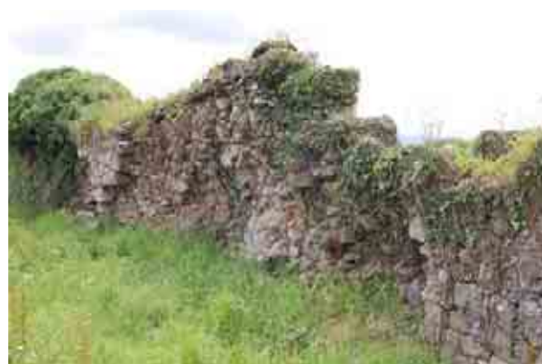
Interior face of Town Wall, with exposed rubble core, looking south-west
