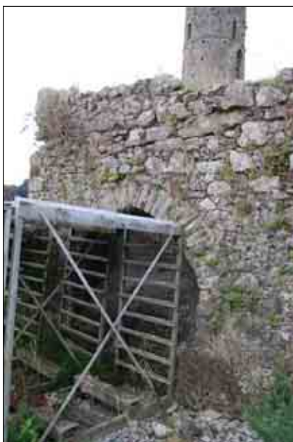
Exterior side of arch, looking south-east
