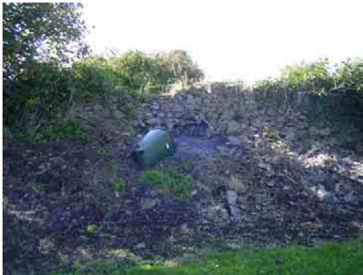
Plate 10: Build up along internal wall face
