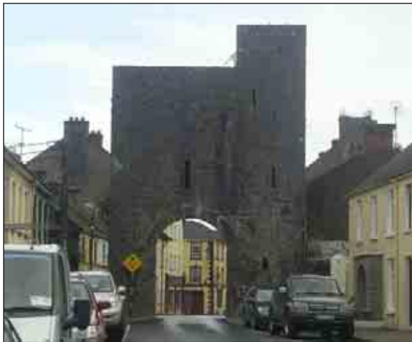
External face of Blossom Gate, looking east
