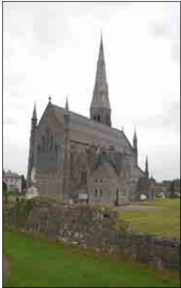
Church of SS Peter and Paul, looking north-east
