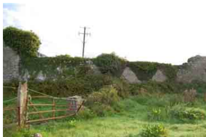
Lower section of Town Wall to south of angle, looking east
