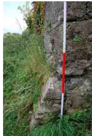
Dressed stones at corner of batter, looking south
