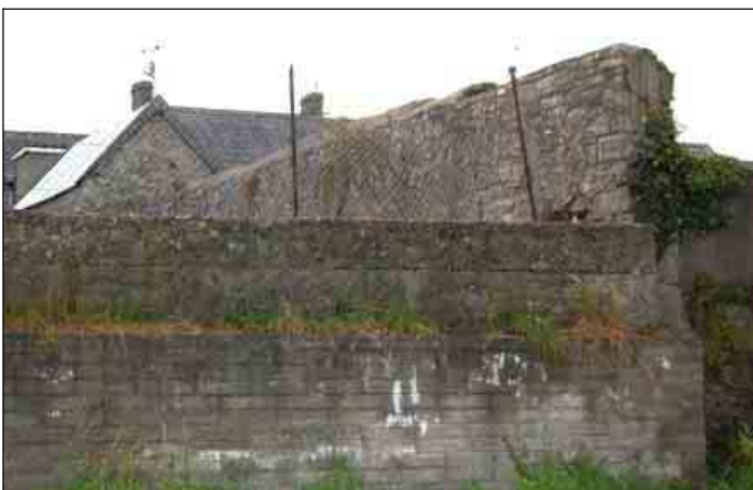
East-west boundary wall at junction with Town Wall, looking south-west
