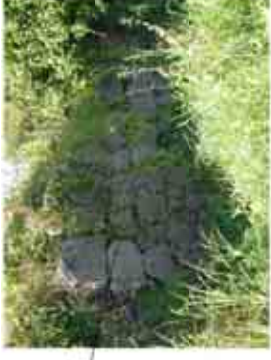
VEGETATION GROWTH ALONG WALL TOP. EXTENSIVE LOSS TO INFILL STONE AND POINTING. (B)
