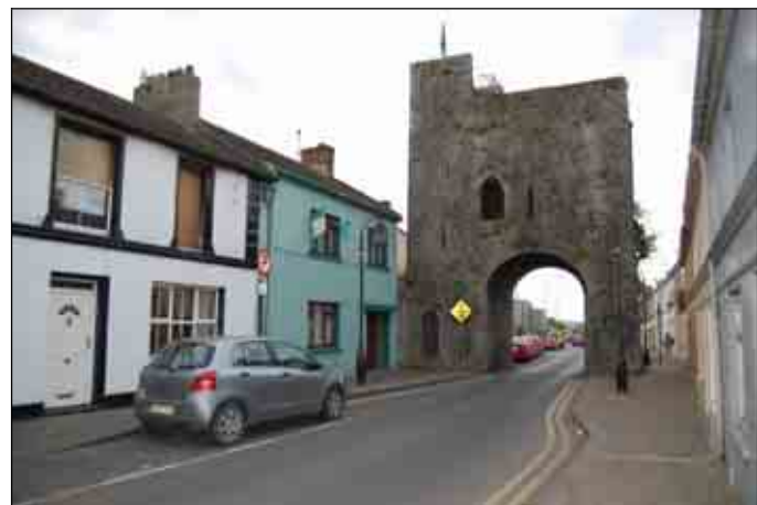
Internal face of Blossom Gate, looking south-west
