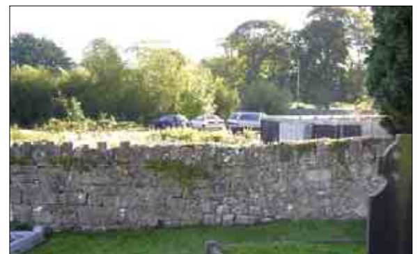
Repaired section of east boundary wall towards south end, looking east
