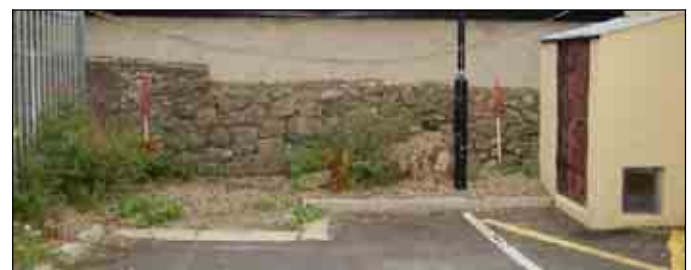
South-west end of wall, looking north-west
