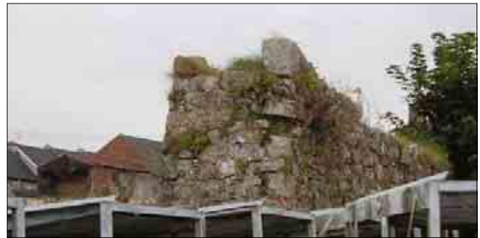
Exterior face of wall above archway, looking west
