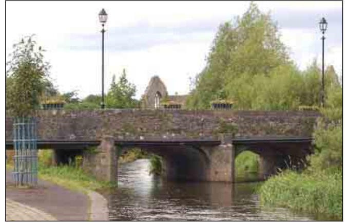
South face of bridge, looking north
