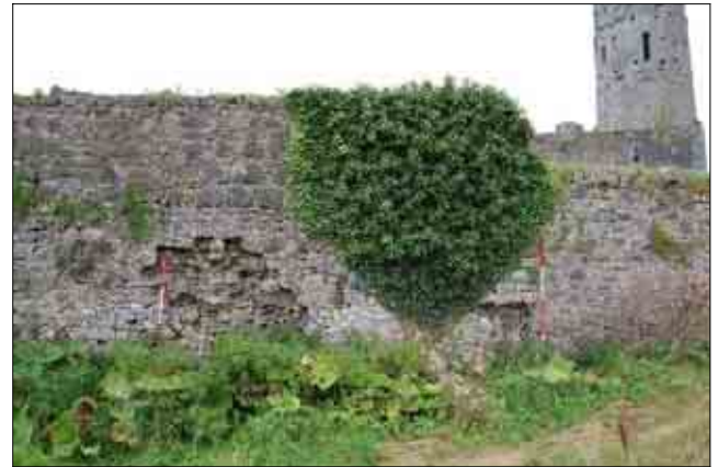
Exterior face of north boundary wall, looking south
