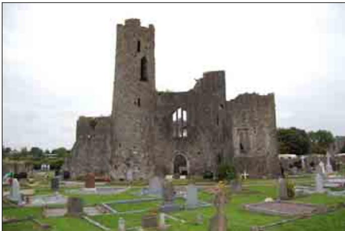
West face of Collegiate church, looking east
