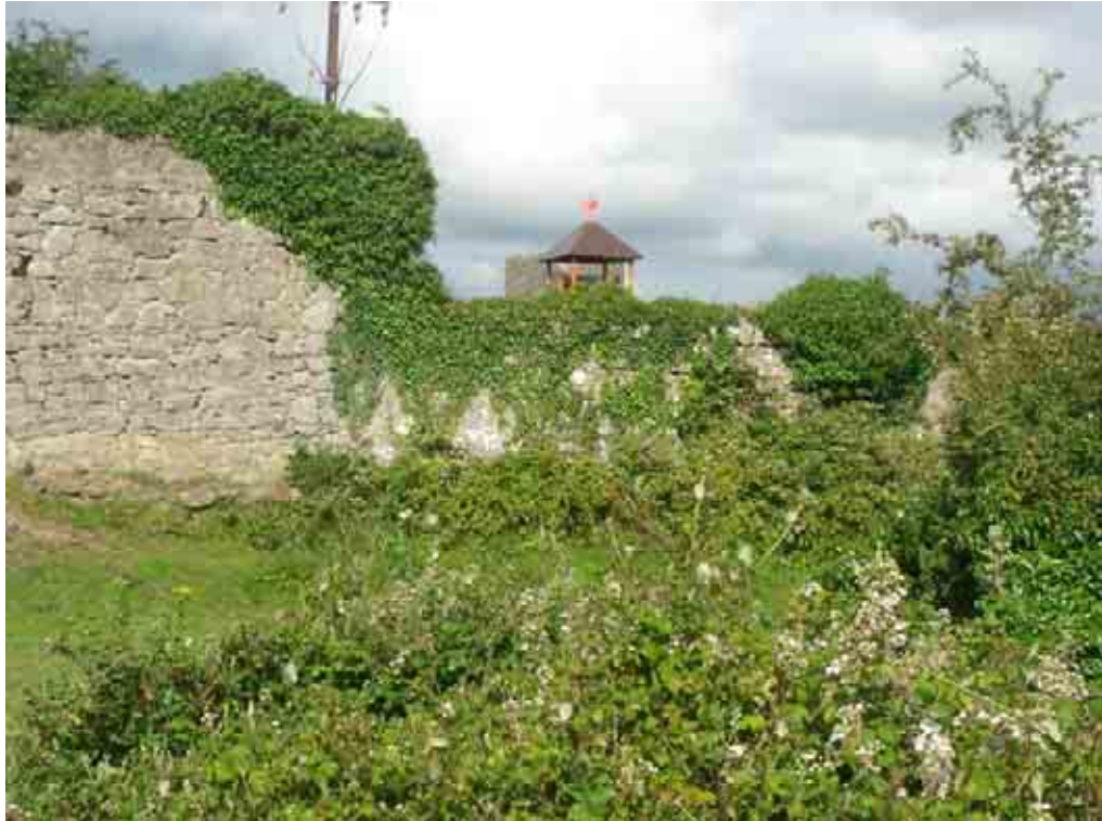
Plate 23: West wall (exterior)
