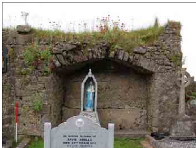
Archway in north boundary wall of Collegiate Church, looking north-west
