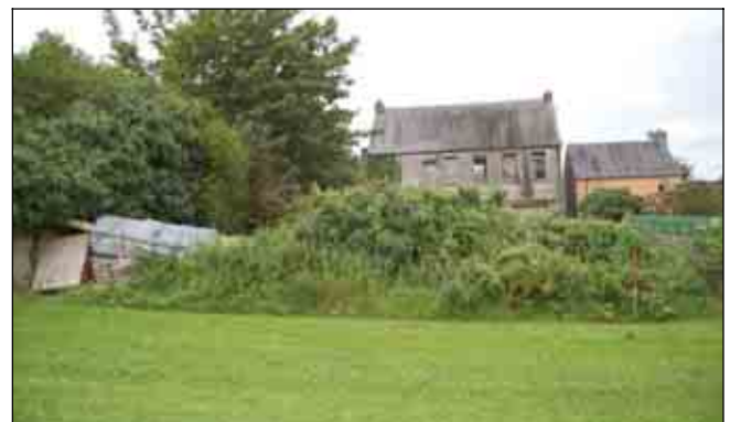
North-east end of wall, overgrown, looking north-west
