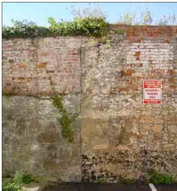
Exterior face of wall, looking north-west
