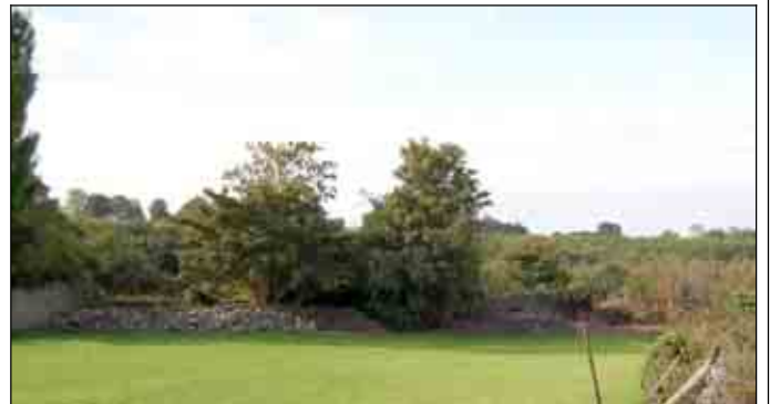
Internal face of Town Wall, north of the stables, looking west
