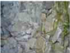
PHOTO 64 & 65. LOSS OF FACEWORK UP TO 350 THICKNESS LOST. CORE REVEALED. URGENT CONSOLIDATION REQUIRED.
