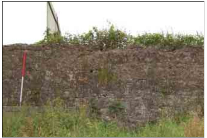
Section of Town Wall along school boundary, looking south
