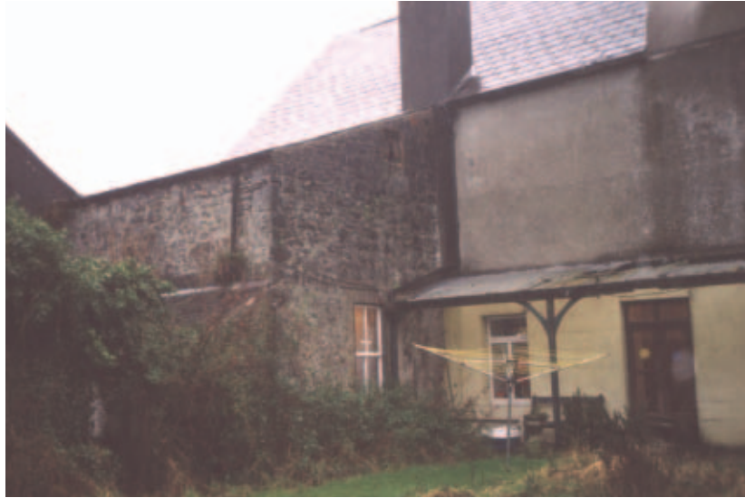
Plate 24: The exterior of Black Rath's Castle
