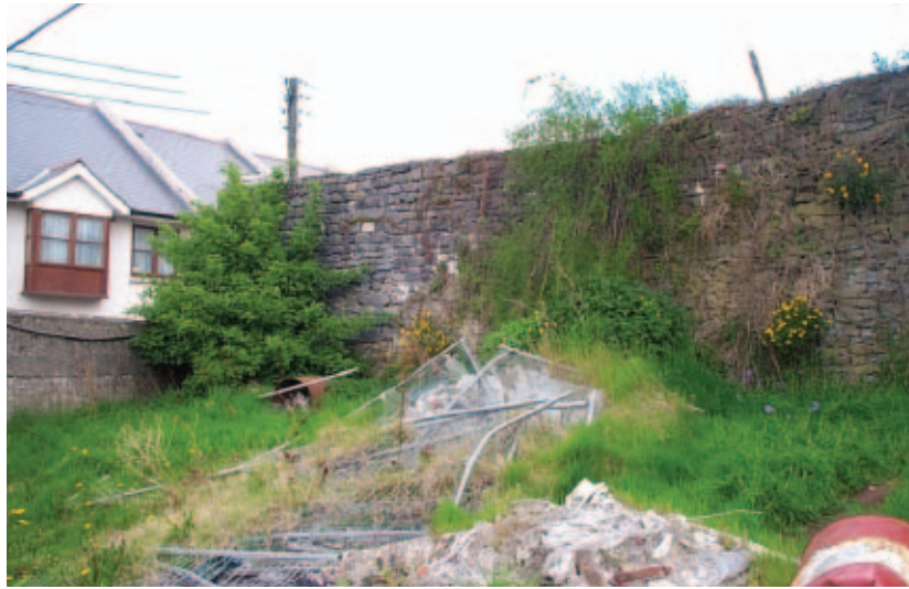
Plate 6: The northern end of the wall is heavily overgrown with elder and sycamore
