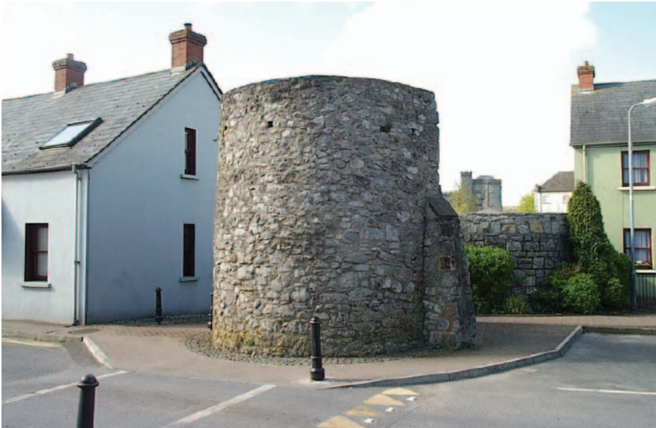
Plate 30: Corner tower from the north-east (May 2001)
