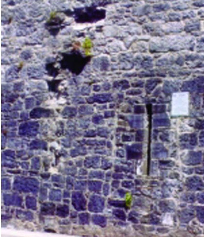
Plate 33: Scar in the south wall of Maudlin Castle, indicating the position of the attached gate (June 2001)
