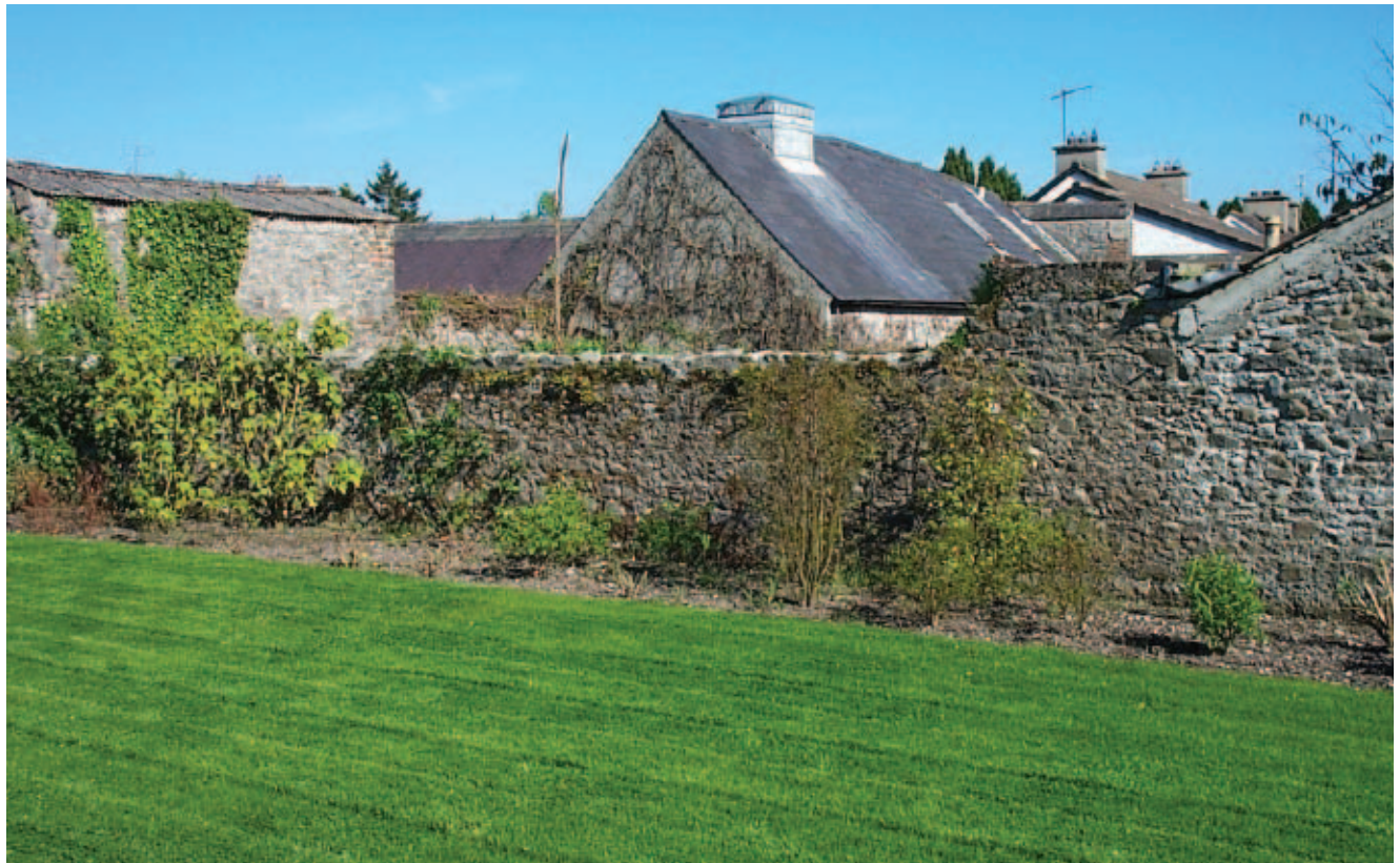
Plate 18: City Wall viewed from the north-west (interior) (May 2001)
