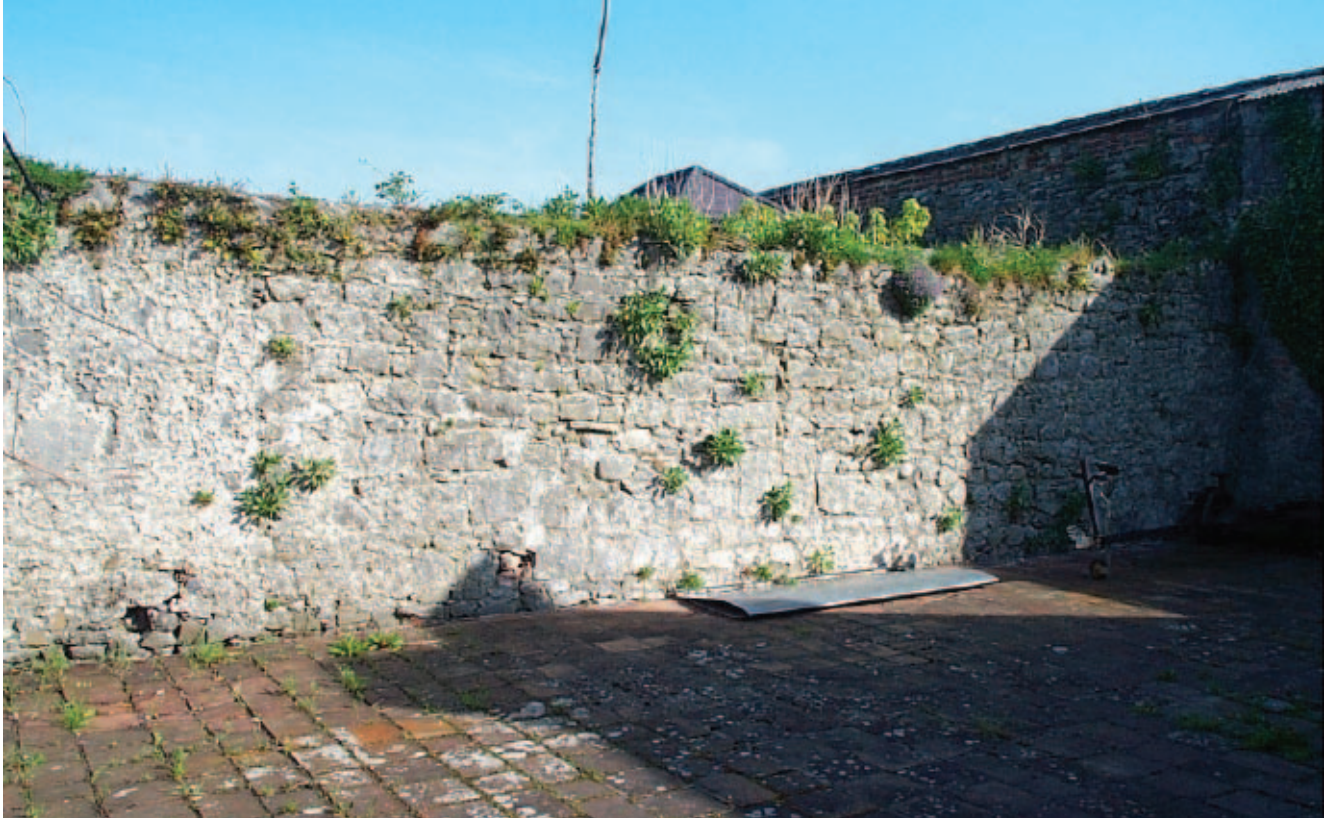
Plate 17: City Wall viewed from the south-east (exterior) (May 2001)
