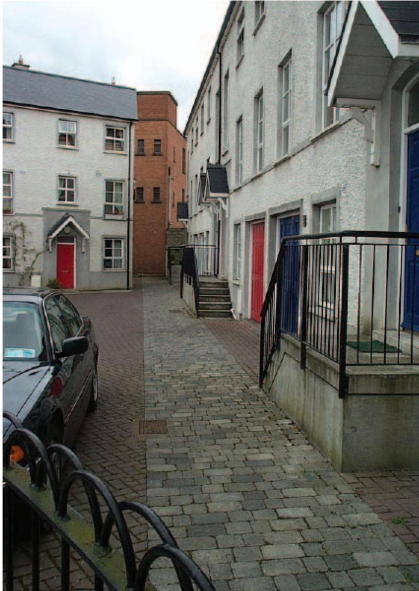
Plate 14: Line of City Wall delineated in grey stone paviours, Ormonde Road (May 2001)
