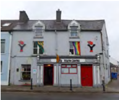
Castleisland project - before
