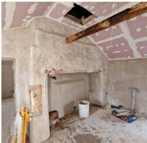
Interior of Goggin Cottage, lime rendering in process – not a straight line in sight! Note area beside chimney where the original layers of lime render have been left exposed.
