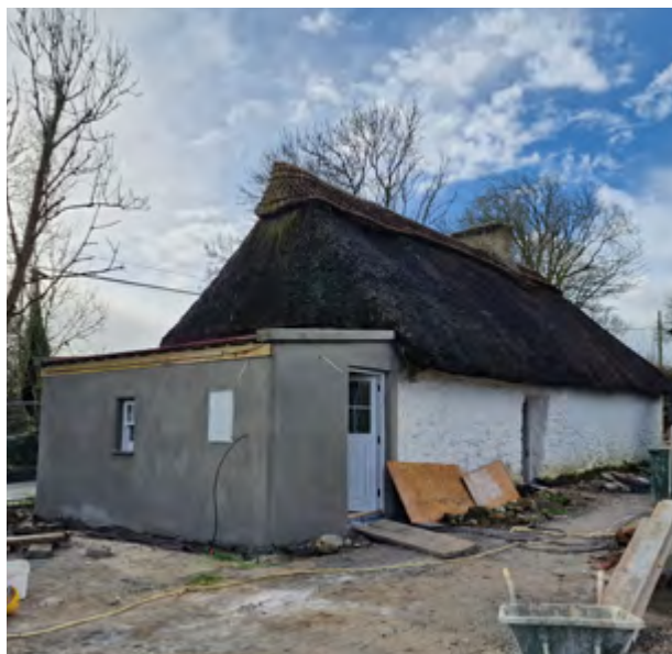
Exterior of Goggin Cottage in February 2024, the former 'lean-to' has been repurposed as a bathroom and utility room for the cottage.
