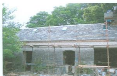
Reinstated rooflights
