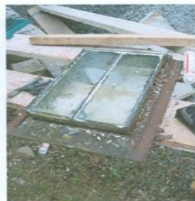
Rooflight being cleaned down
