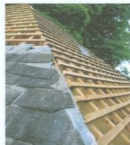
Existing light weight rafters predominately retained with new 3"x2" battens screwed to topside to improve rigidity and framing.
