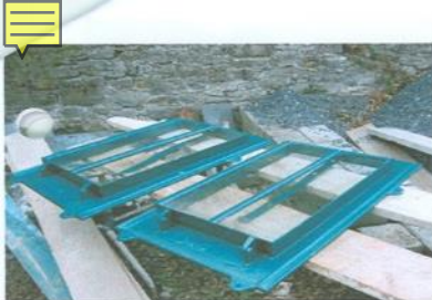
Cast iron rooflight units being re painted
