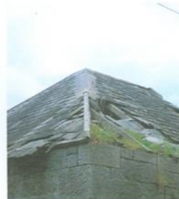
Lead roll hip detail from shed B to be used as model for shed A
