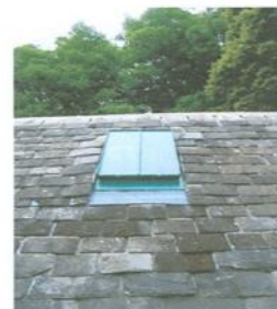
Completed rooflight in-situ
