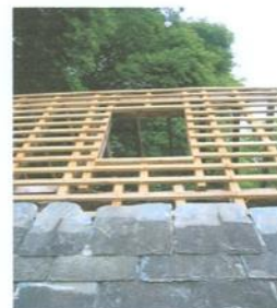
Existing rooflight opening being prepared for reinstatement of rooflight frame
