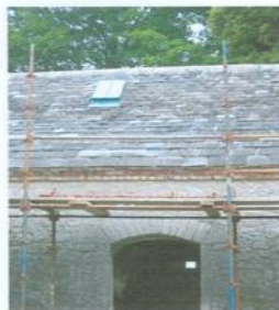
New slating graded to match original
