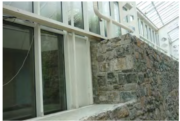
Fig.86 Detail of steel framework to top of wall head.
