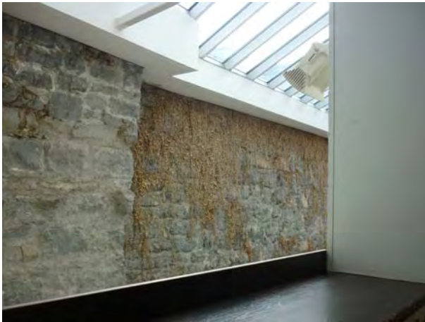
Fig.37 Detail of glass roof on top of wall at Eyre Street
