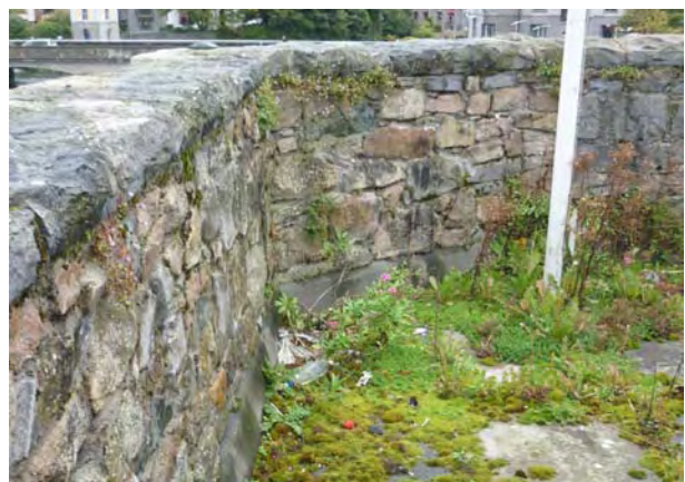
Fig.56 Detail of poor drainage to wall walk at Spanish Arch.
