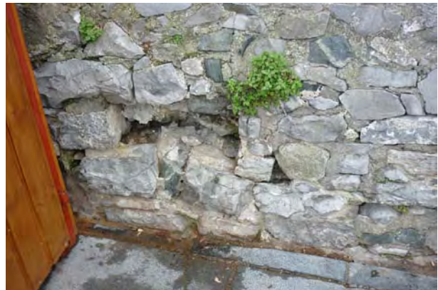
Fig.55 Detail of stone damage at base of Spanish Arch.
