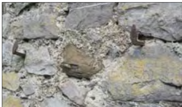
Plate 50: Detail of historic metal fixings in south wall at St Mary's. Note also original lime mortar
