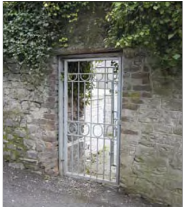
Plate 26: Inappropriate repairs at doorway and corroding metal lintel Featherbed Lane
