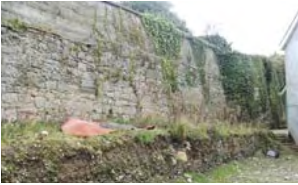
Plate 12: Rear boundary wall, 98 George's Street. Note the curve in the town wall, reduced ground level and new development close to town wall
