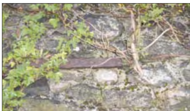
Plate 46: Metal ties, vegetation and poor point-ing at St Mary's
