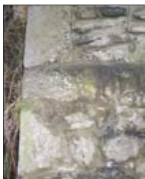
Plate 47: Cementitious pointing "battered" on to stones at St Mary's
