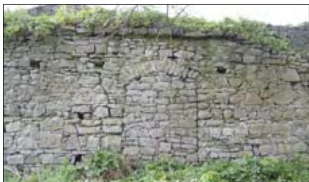
Plate 43: Open joints, deteriorated coping and vegetation at St Mary's "blind" gate. Note gaps in stonework are Putlog holes used for scaffolding the wall when first built
