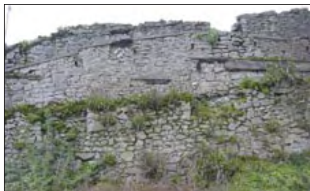
Plate 7: Line of wall-walk at Murdock's Yard car park. Note also timber inclusions and cement eaves of former lean-to buildings
