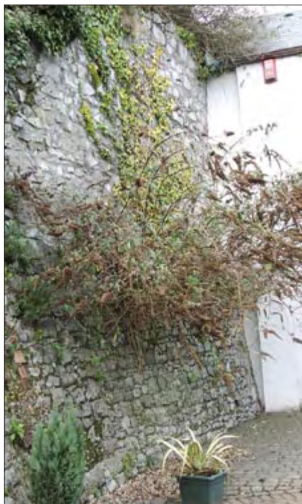
Plate 28: East face of Featherbed Lane. Vegetation grows at the top of the batter and in line with ground level on the western side of the wall.
