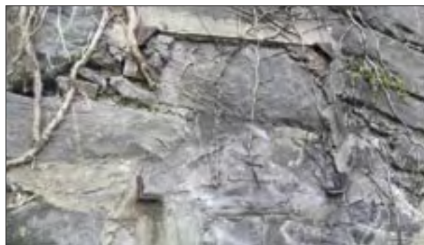
Plate 68: Metal inclusions, inappropriate repointing and vegetation at Butter Gate
