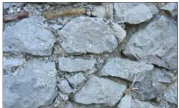
Plate 63 Construction join west of Millmount. Note the two different mortars used.
