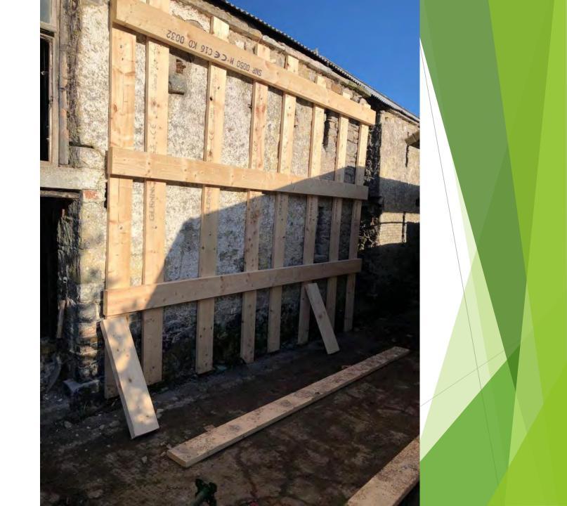
Internally the existing roof was jacked to its original position using a system of raking 9" x 3" timbers which were jacked received distance in the position of the wall opposite. Following this wall was gradually jacked in position using two taps of a sledgehammer at each jacking point in rotation. This was carried out under the careful supervision of Chris Southgate. The wall was able to realign to its original position.
