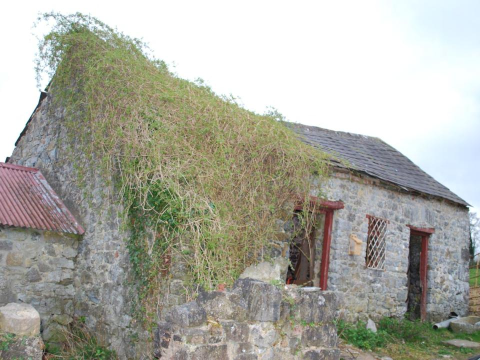
The roof had literally pushed walls outwards causing major cracks in the gable walls
