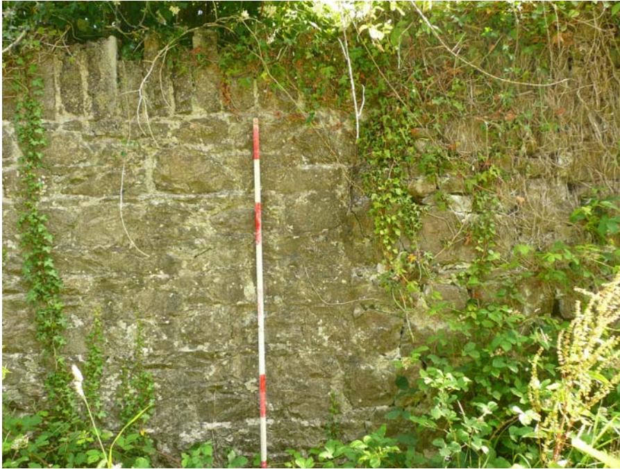
Plate 5: Wall on north side of Mill Lane. Note break in construction styles to right of ranging rod. Older wall to right, modern wall to left.
