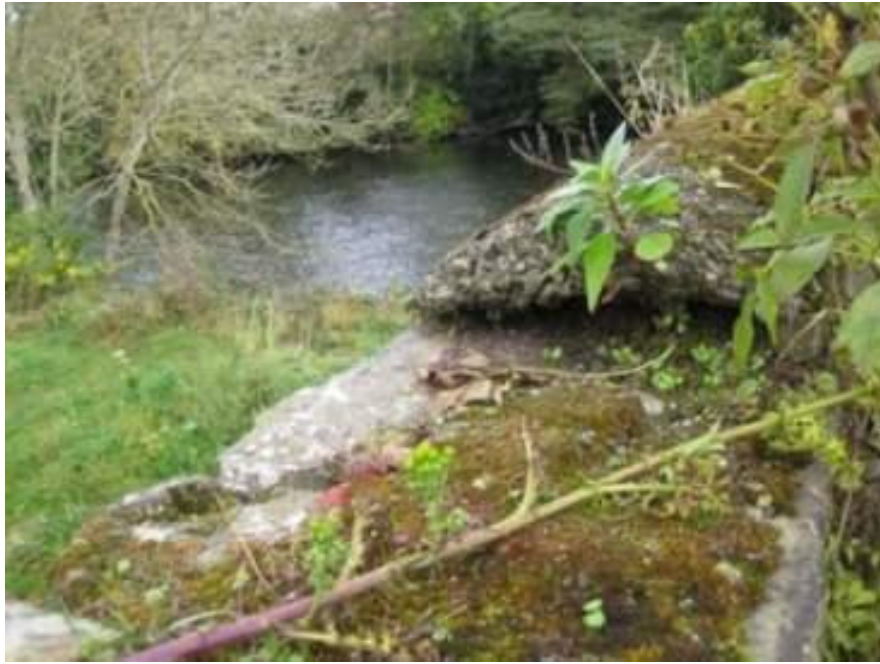
Plate 57: Damaged flaunching to west wall
