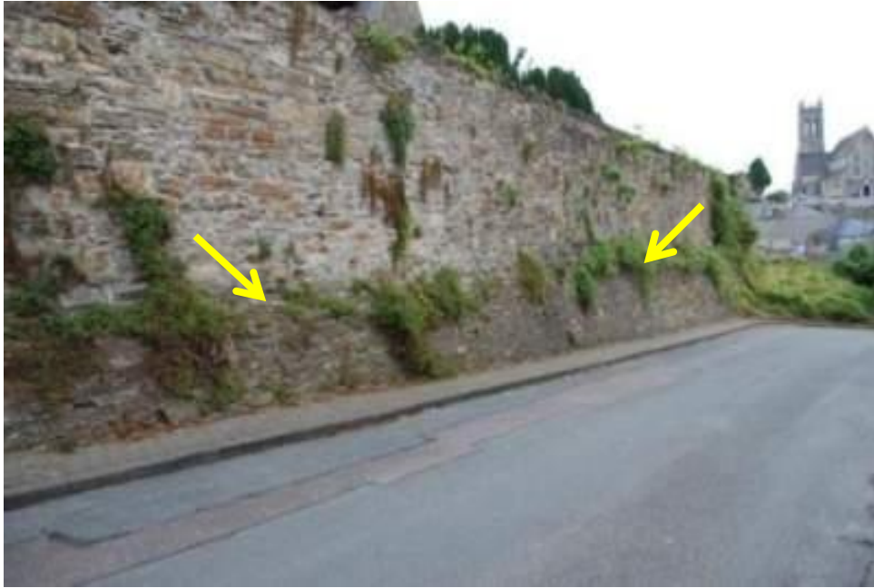
Plate 20: Original base batter visible on south-facing elevation of Section 5. Rebuilt wall on top of batter forms southern boundary of St Peter's graveyard.
