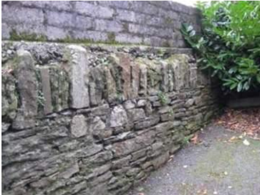
Plate 81: Open joint to Section 10.
