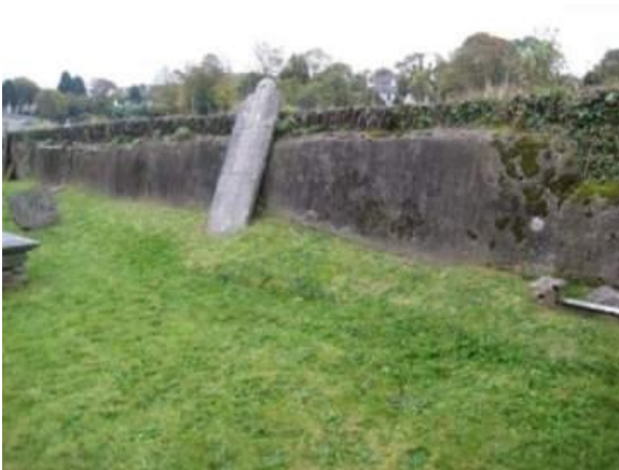
Plate 68: Cementitious render to north elevation
