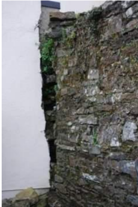
Plate 8: Original town wall (east elevation) where it is abutted by shopping centre building – note collapsed masonry.
