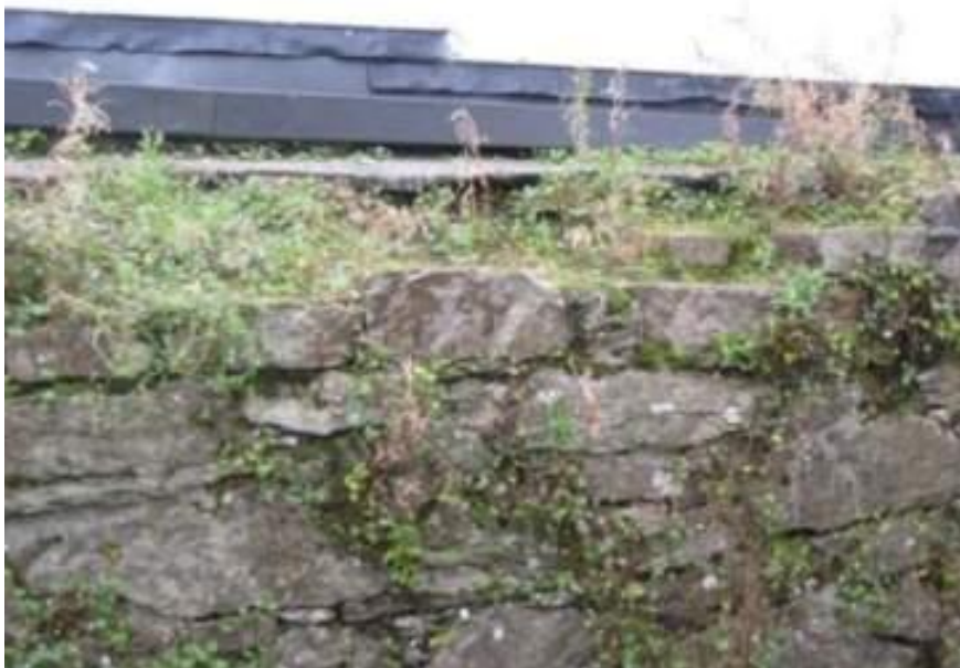
Plate 63: View of section beside Riverside Shopping Centre showing damaged coping and biological growth
