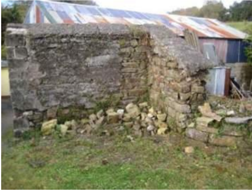
Plate 91: Concrete render to potential structure
