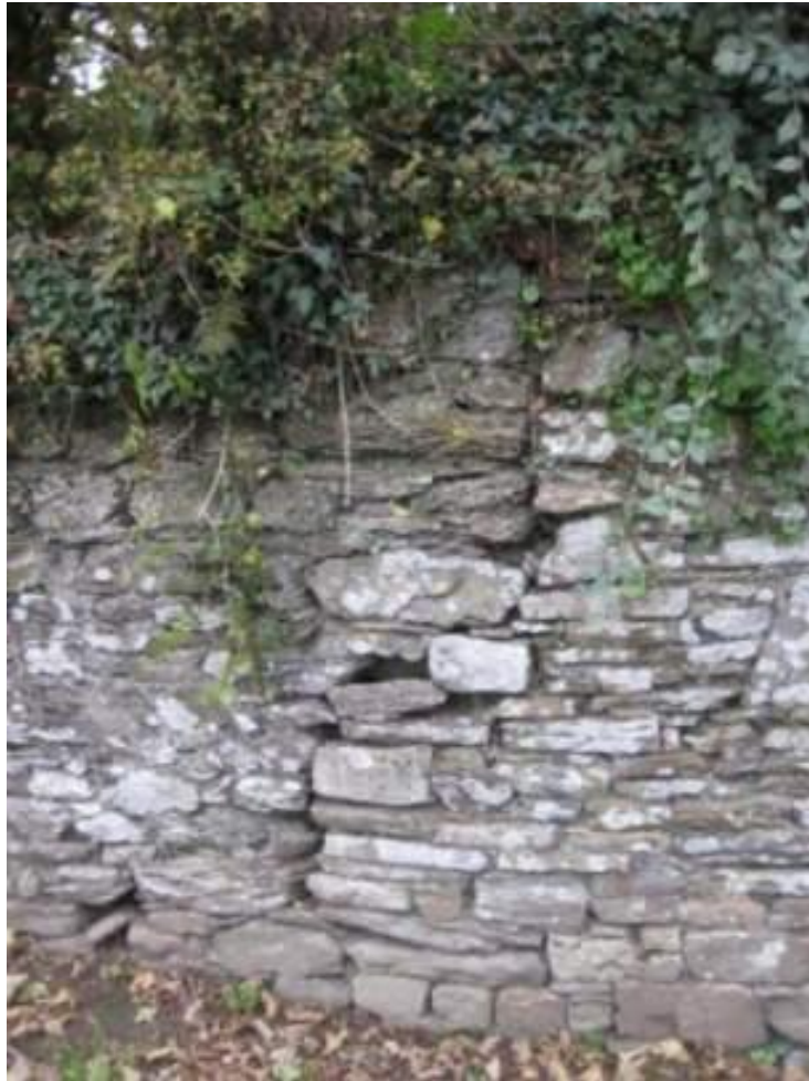
Plate 77: Crack to south elevation of wall
