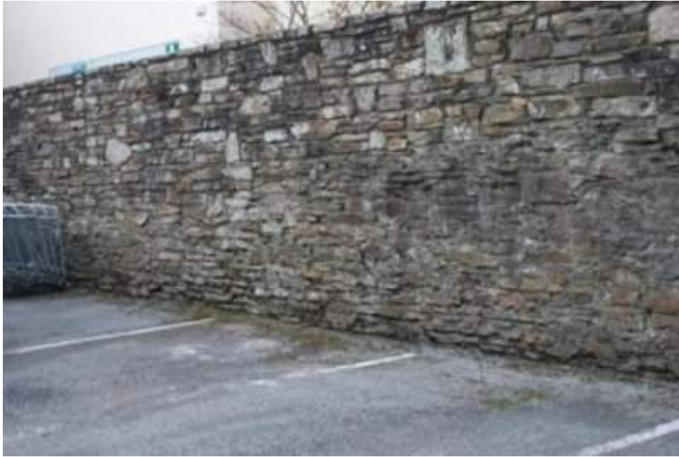
Plate 7: Original wall surviving to varying heights beneath modern rebuild (East elevation).
