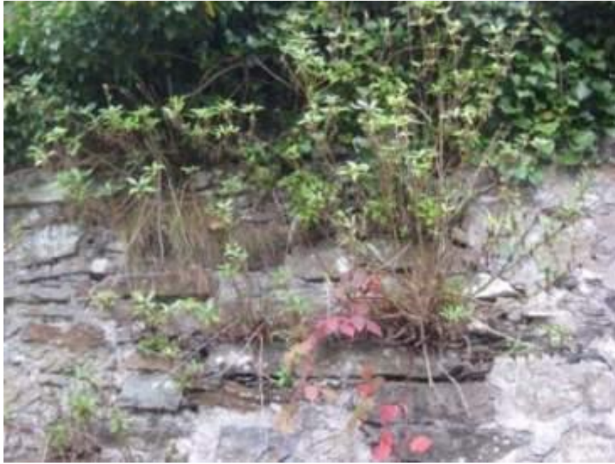
Plate 72: Open joints to wall which have encouraged the growth of plantlife
