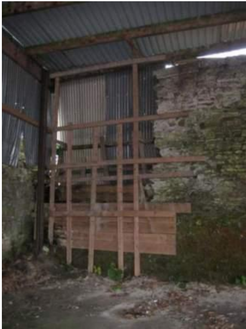
Plate 87: Breach in east-west running section of wall. Note growth of moss to lower reaches of wall
