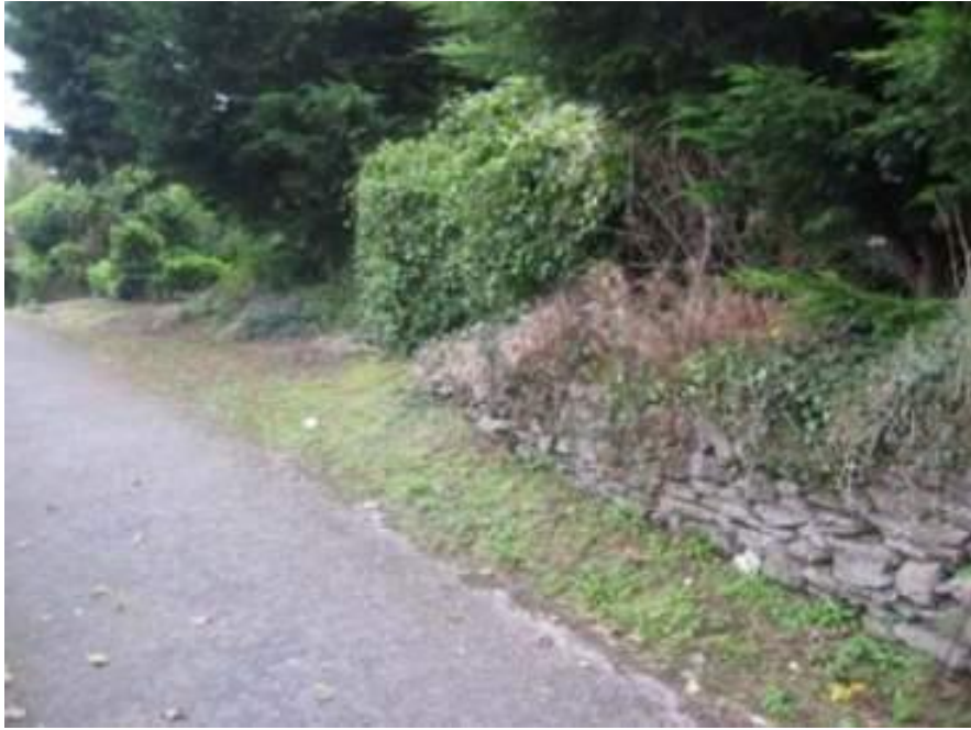
Plate 75: View of wall from southeast showing biological growth, open joints and general poor state of preservation of wall
