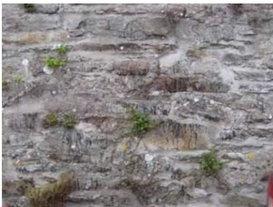
Plate 71: Biological growth and bitumen residue to wall
