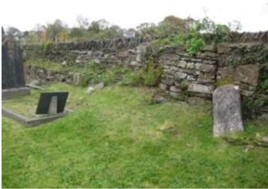
Plate 67: North elevation of wall showing open joints, loss of fabric and biological growth
