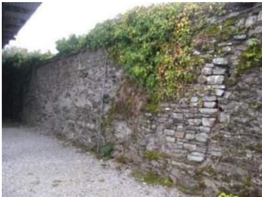
Plate 86: View of wall southwest showing vegetation growth and evidence of rebuilding of wall
