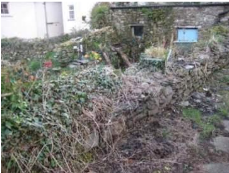
Plate 92: View of section of wall from northeast showing vegetation growth, loose stone and open joints.
