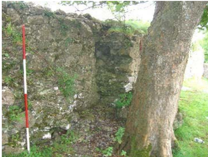
Plate 8: Breach rebuilt in stone, but to a lesser thickness
