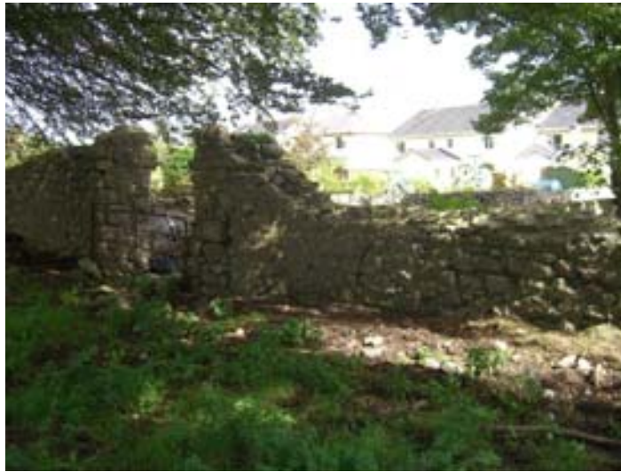
Plate 10: Unprotected wall tops
