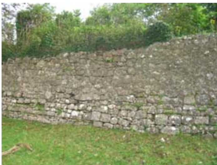
Plate 7: Typical elevation showing random coursing, galleting and open joints near the base
