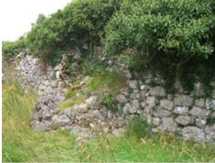
Plate 9: Collapse of wall face
