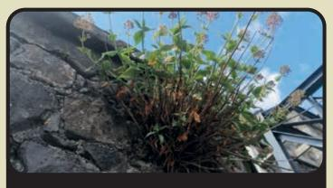
The Valerian is opening up masonry joints, allowing water ingress and creating a localised bulge.
